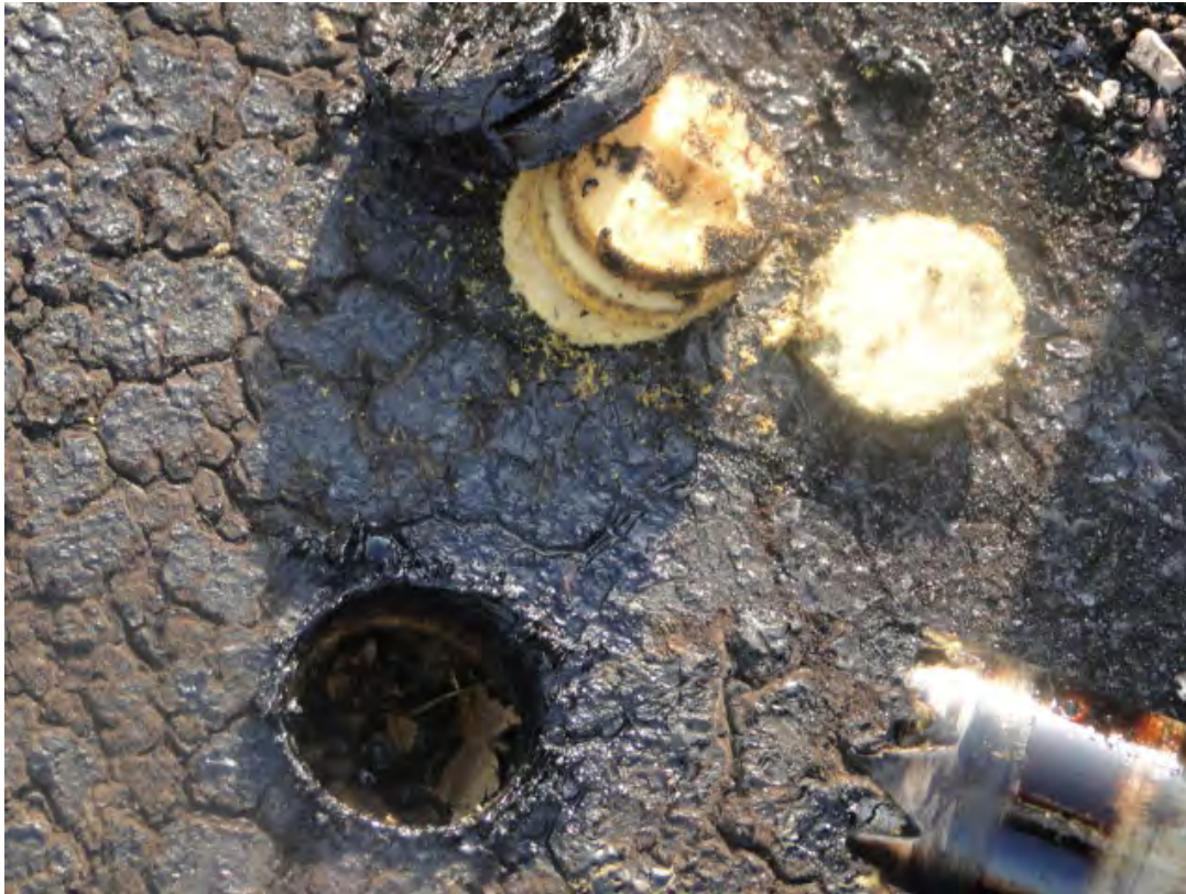
Photo #3 View of roof core cut at Bldg. B006.
