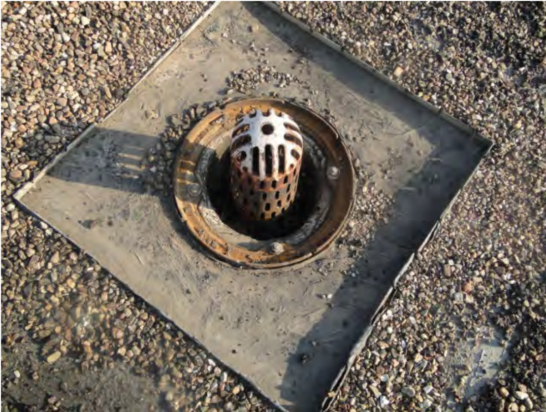
Photo #5 View of existing roof drain at Bldg. B006.
