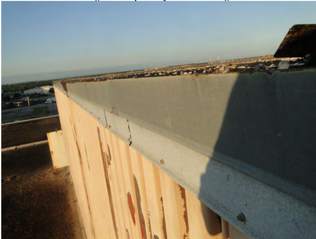
Photo #16 View of existing metal fascia at Bldg. B116 penthouse.
