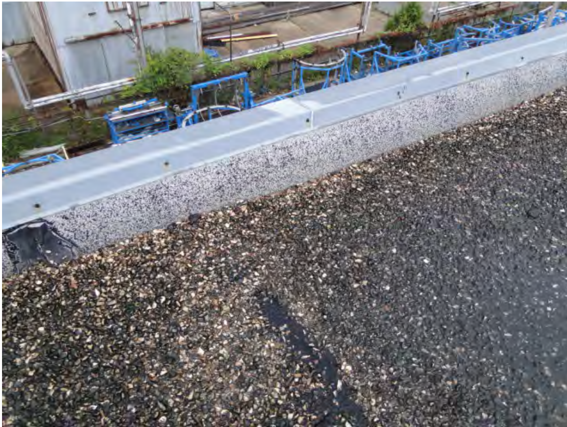
Photo #13 View of existing metal coping at Bldg. B116.
